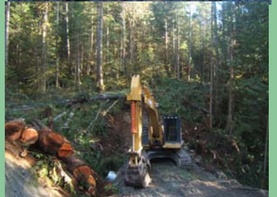
Examples of high-quality road construction practices were observed in the field.
