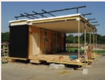
**SFI program participants donated wood products for the construction of North House. The photo shows preliminary testing and dry-fitting of the rooftop truss assembly.**
